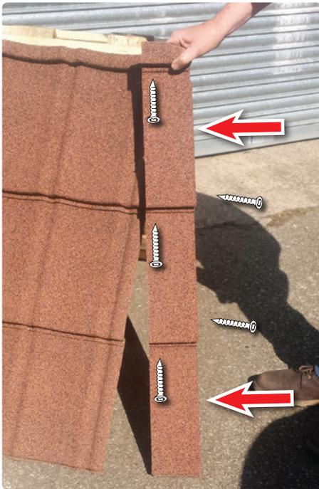
Screw through the dry verge into the battens as pictured. **Three** in each tile overlap and **two** on the front edge, ensuring the screws penetrate the framework.
