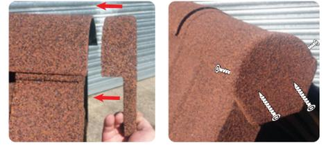
Screw through the end cap AND ridge tile into the batten. Optionally, screw through the face of the end cap, through the dry verge and into the batten.
