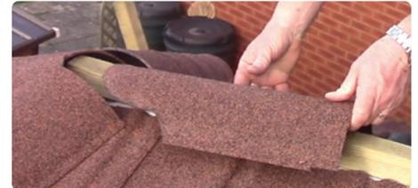
In some cases, Lead or a Lead Alternative such as Ubiflex can be used to create a water-tight seal (Cap). The picture below shows fitted cap (*not supplied*).
