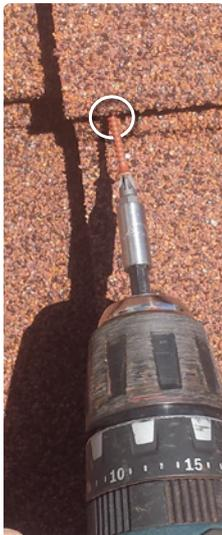
**TIP:** Always insert the screws into the overlap.
