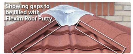
Showing gaps to be filled with Flexim Roof Putty
