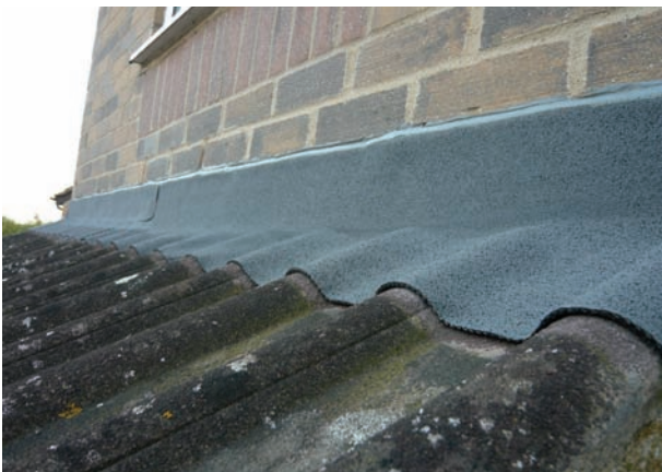
Flashing to a domestic entrance porch
