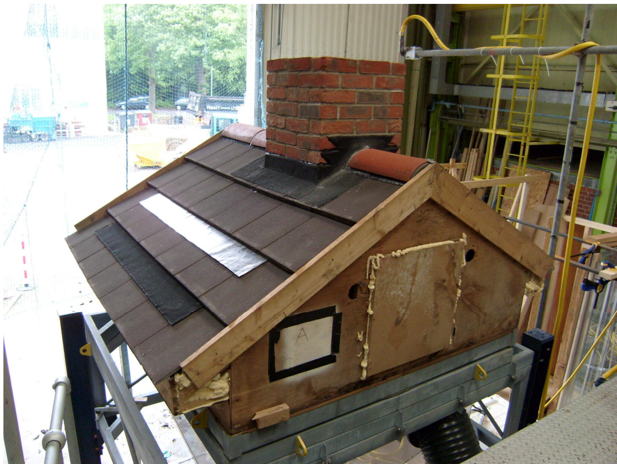
Figure 2. Side 2 Flat concrete tiles and flashing around chimney with additional flashing fitted between courses of the roof tiles.
