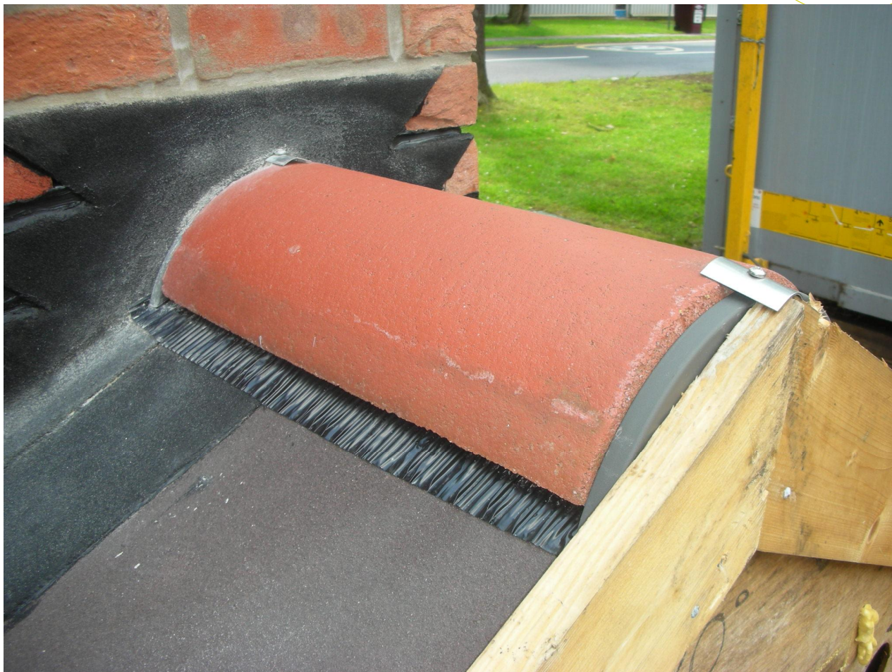
Figure 3 Side 2 showing detail of the Ubbink Ventilated Dry Ridge system
