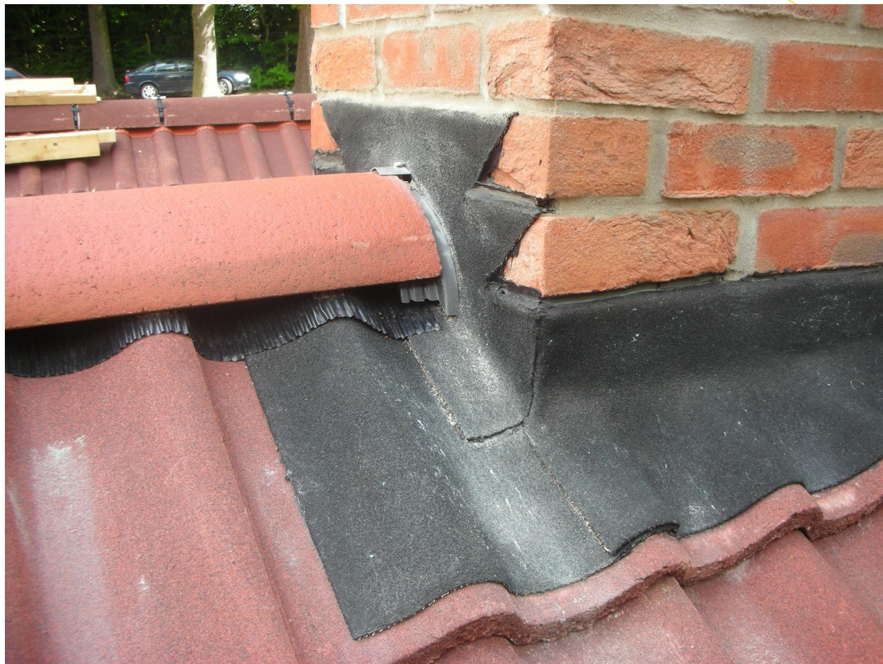
Figure 4 Side 1 showing detail of Ubbink Ventilated Dry Ridge system
